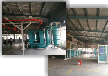
11 Tank Semi-Automatic Powder Coating Plant
