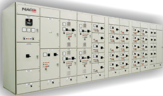
Low Voltage Panel Solutions
